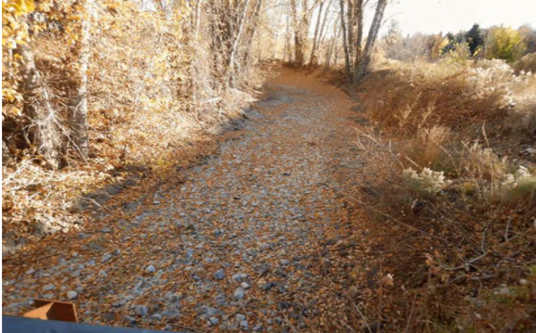
Upstream Channel Looking North
