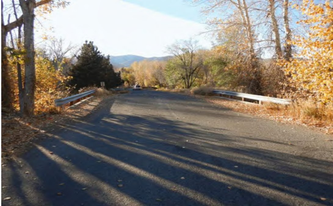
Approach Roadway Looking West
