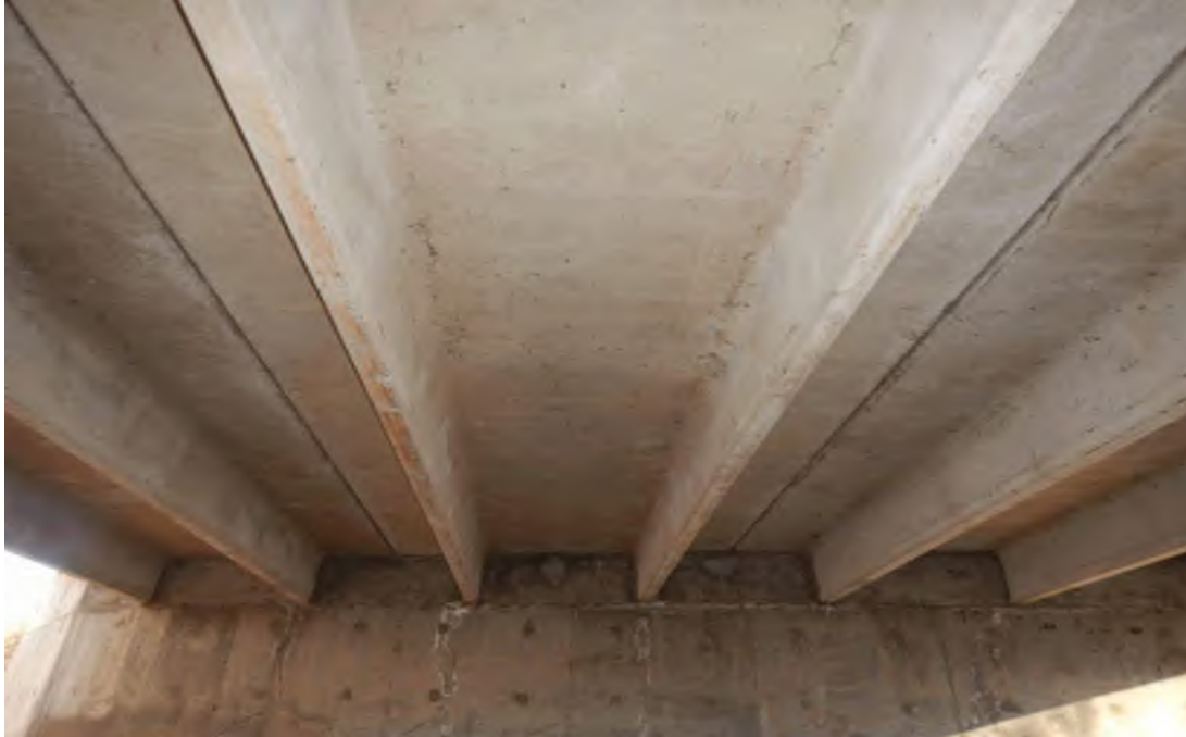
General Underside Condition
