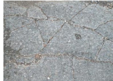
Figure 8: Fatigue Cracking
