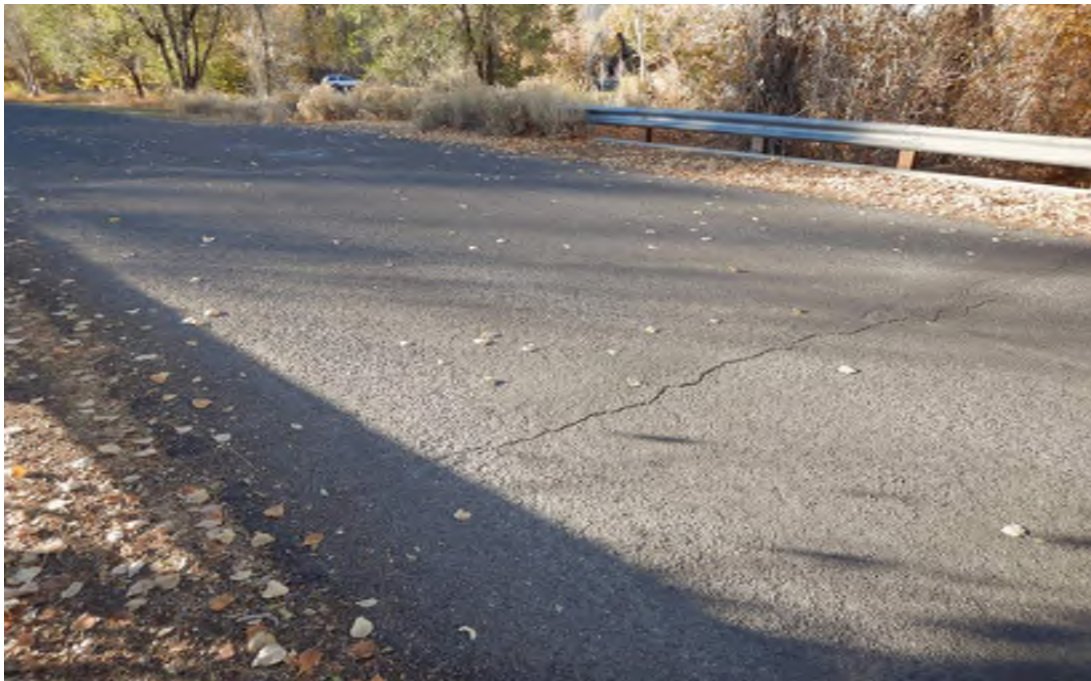
General Topside Condition
