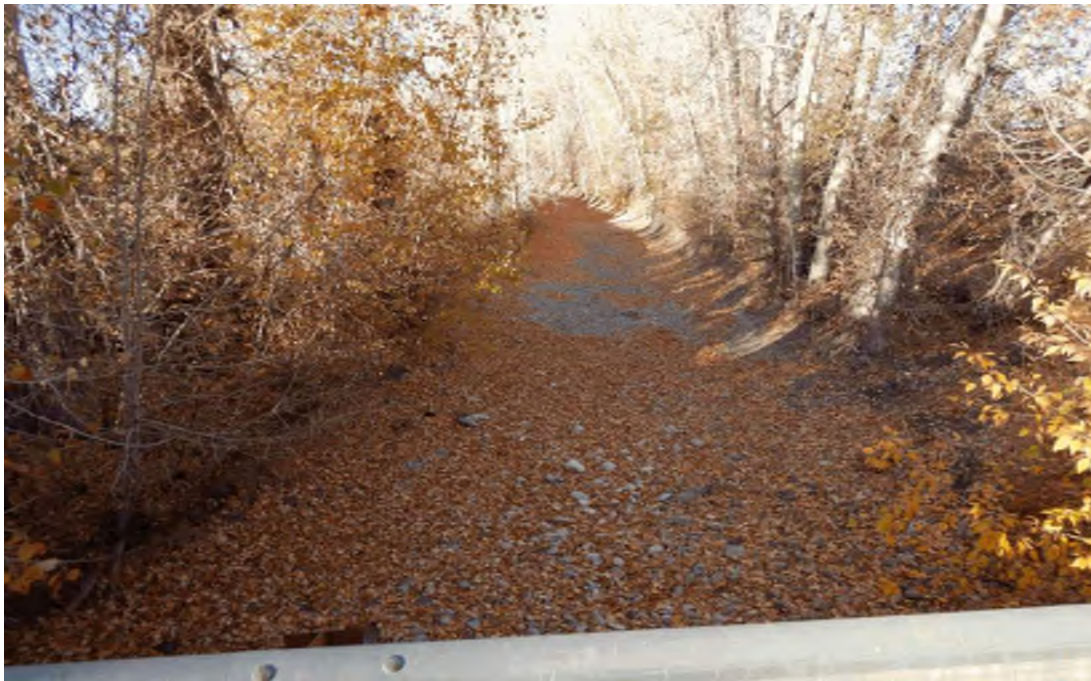
Downstream Channel Looking South
