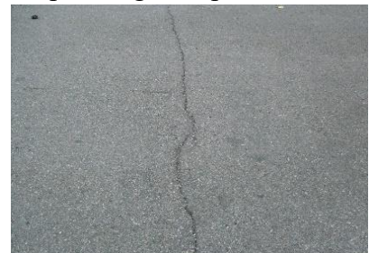
Figure 9: Longitudinal Cracking
