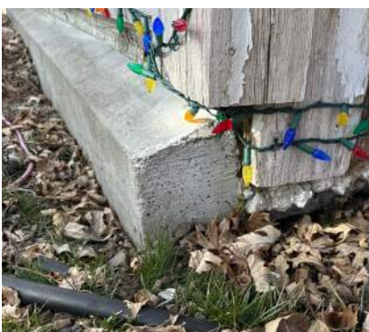
this is what was constructed on the south wall ...
