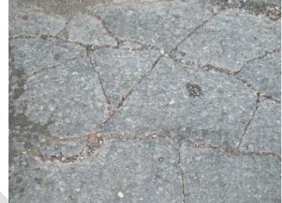
Figure 13: Fatigue Cracking
