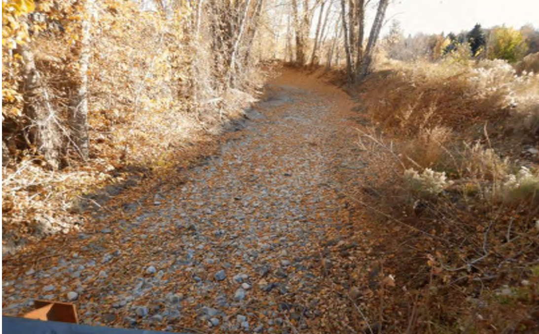
Upstream Channel Looking North
