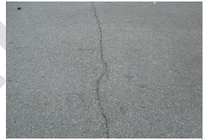
Figure 14: Longitudinal Cracking
