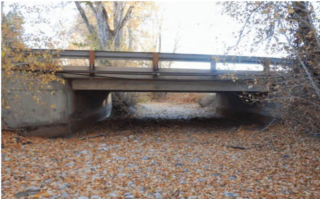
Elevation View Looking South
