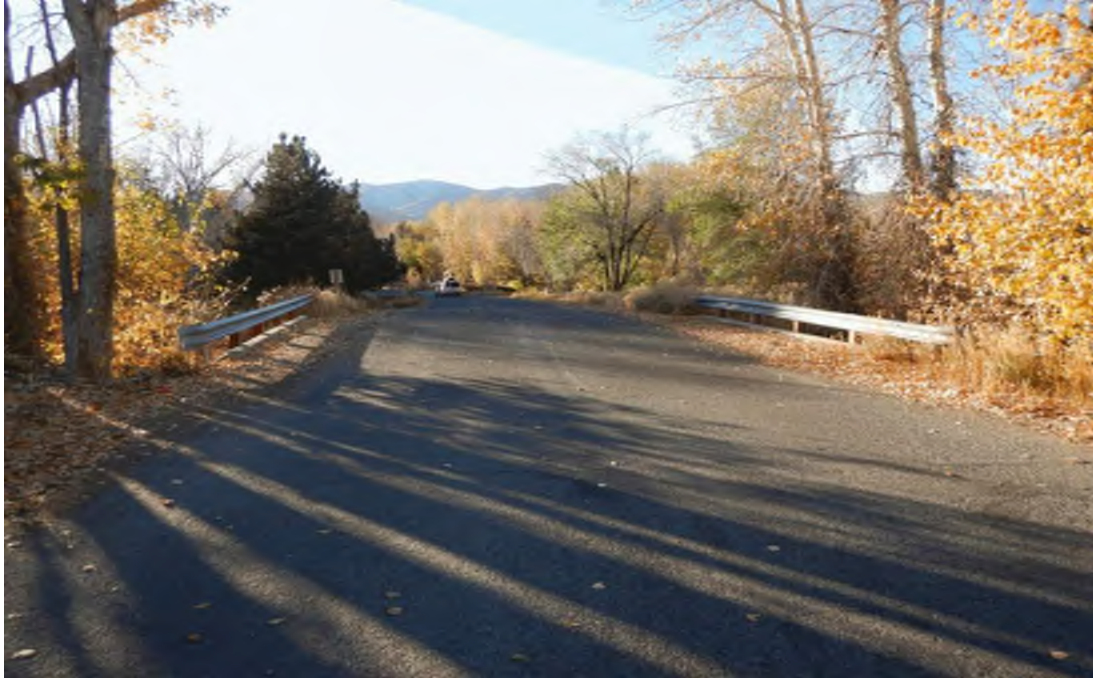
Approach Roadway Looking West
