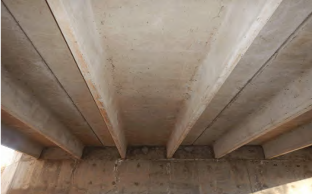
General Underside Condition
