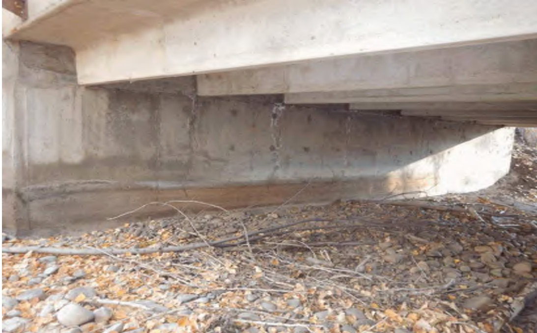
General Abutment Condition
