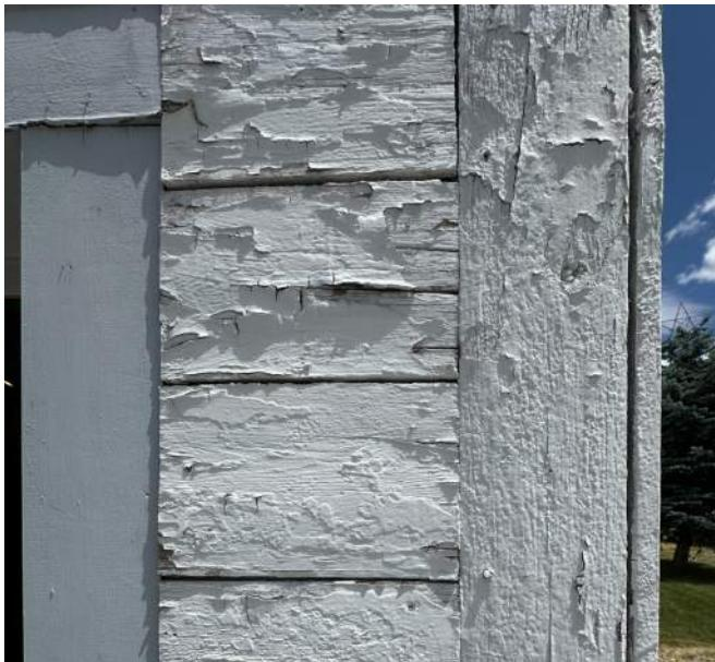
Deteriorating paint on southwest corner of west facade
