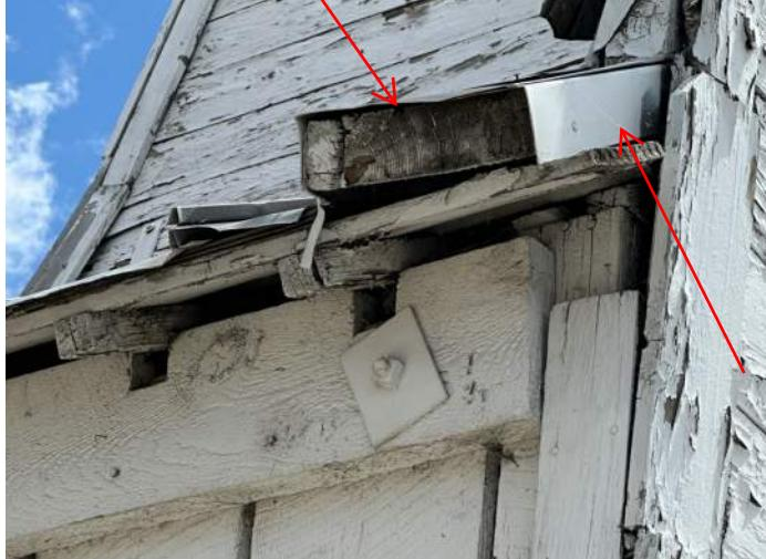
South side of west facade with missing roof covering at corner and exposed rot in gap
