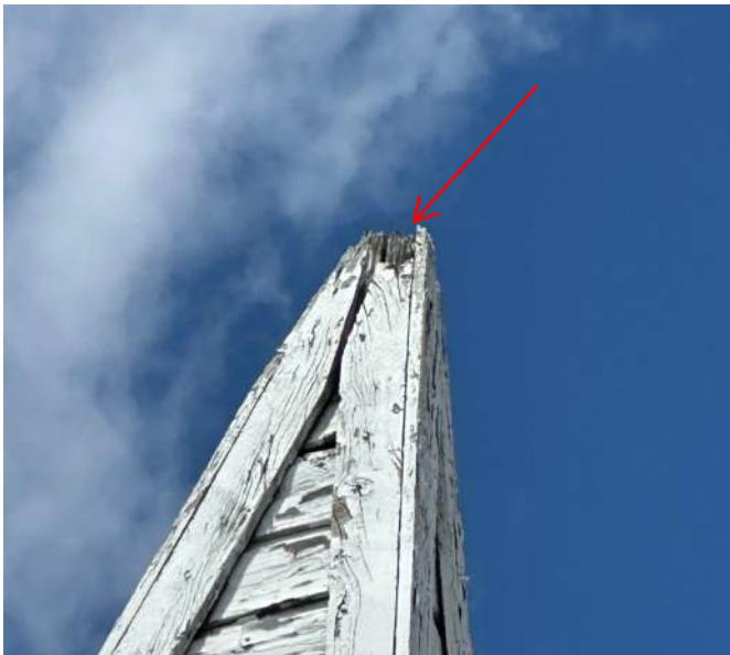
Top peak of bell tower missing any flashing to protect the wood and interior of the structure. Note rot of structure at the top
