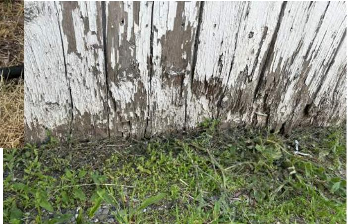
North wall with bottom of plank wall buried in soil
