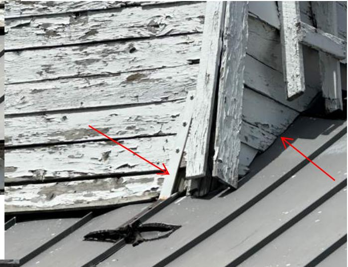
Southeast corner of bell tower. Note suspect connection to the roof, missing flashing, and loose trim boards
