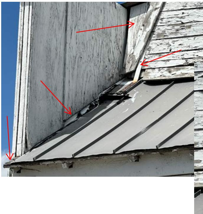
Southwest corner of bell tower and backside of west facade. Note suspect construction to west of bell tower, bell tower attachment to the roof, missing flashing, and exposed roof sheathing at corner.
