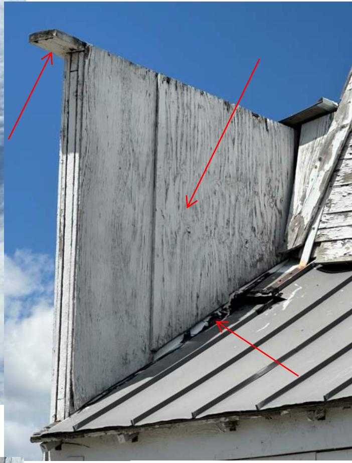
North side of west facade with flat 2x supporting bell tower and missing roof covering at corner
