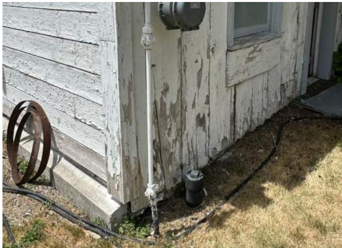
Southeast building corner at grade with gas service and sewer line cleanout. Rot at base of east wall and new concrete curb on south wall. Note also depression in grade that will collect water runoff.
