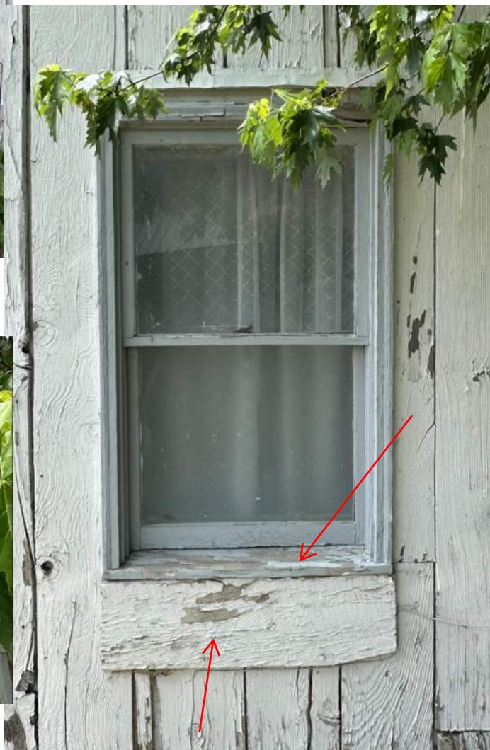
Southeast window. Note rough board sill which should remain. Window sill needs repair
