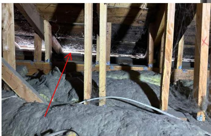
Attic with new structural framing and showing daylight at the gap between wall framing and roof structure
