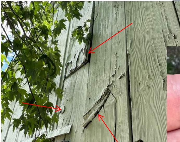
Deteriorating paint, loose plank and knots on east facade
