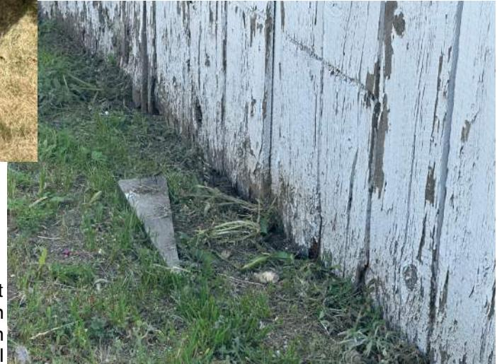
North wall with rot at bottoms of plank wall which are buried in or resting on soil
