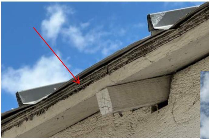
North roof eave with exposed plywood sheathing which should be covered with metal drip edge
