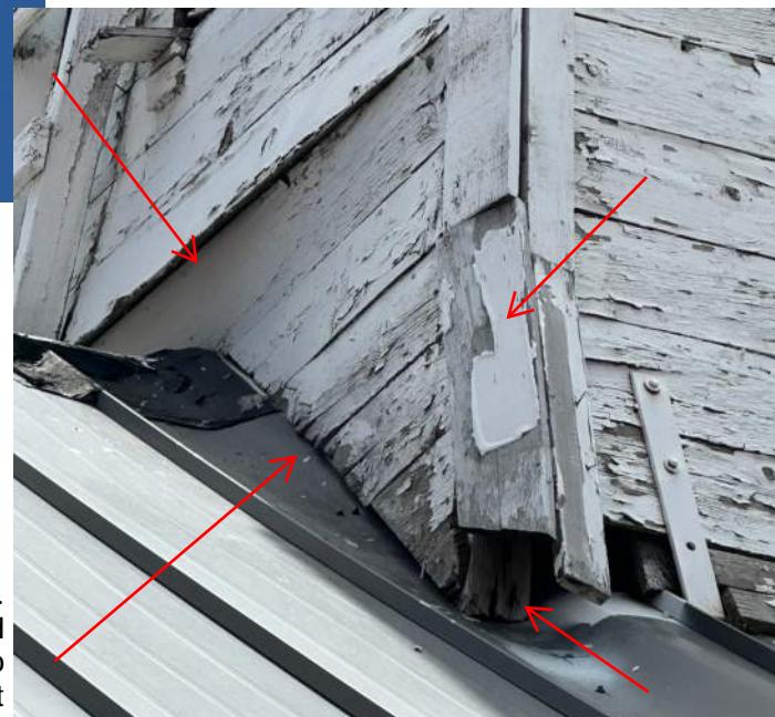
Northeast corner of bell tower at bottom. Note collapsed structure, displaced wood trim (from snow and ice movement), no flashing, and wood rot
