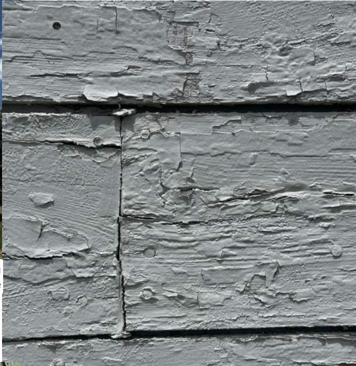
Deteriorating paint on south facade
