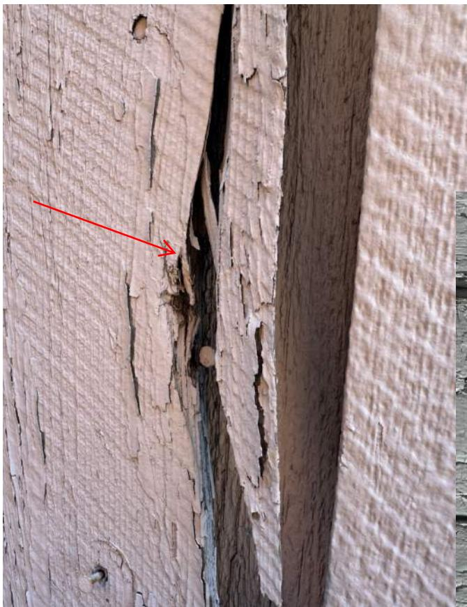
North wall with fractured or split edge of plank construction
