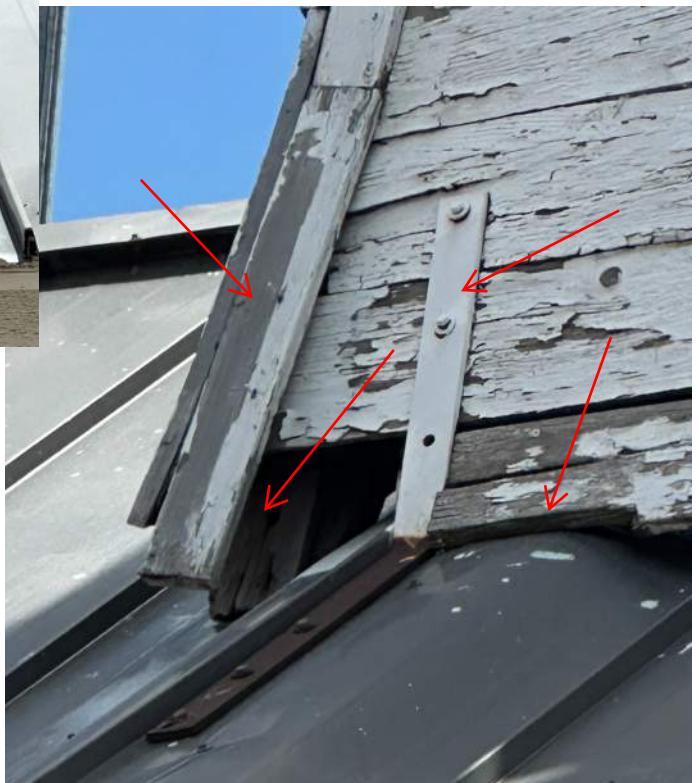
Northeast corner of bell tower with suspect attachment to 2x member (noted previously), wood rot, and damaged trim.
