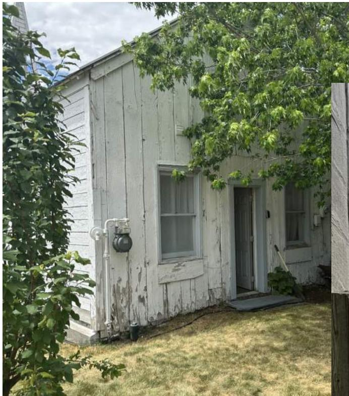
East wall with rot at bottoms of plank wall construction
