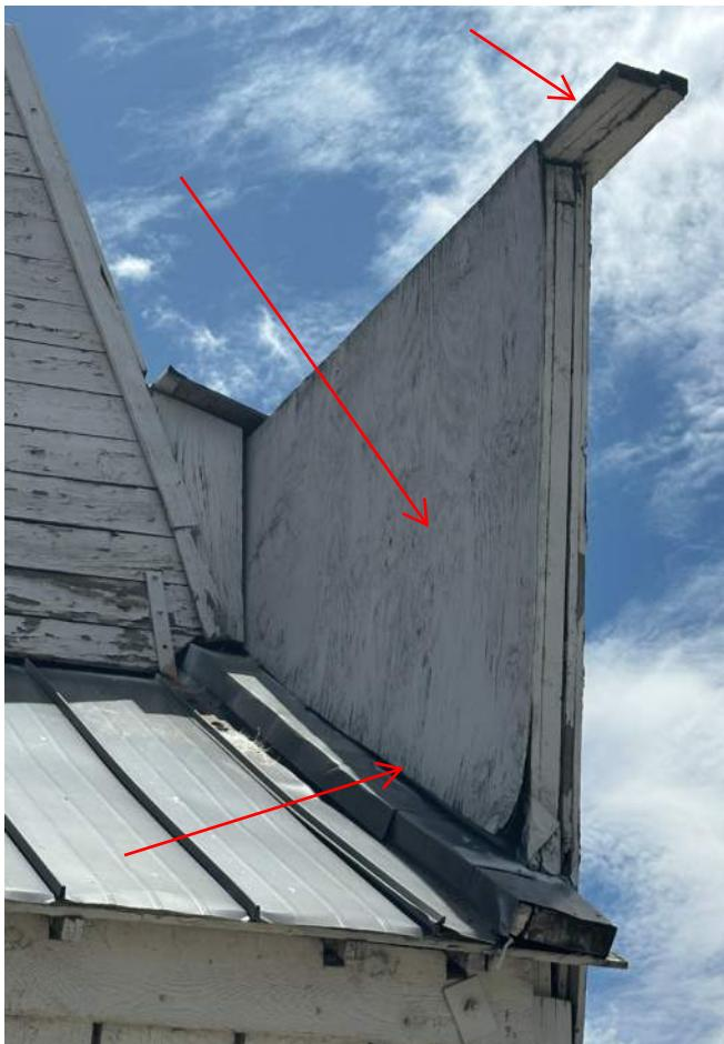
North backside of west facade with plywood, cantilevered exposed board, and missing wall flashing at roof
