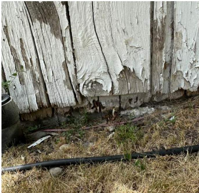
East wall where bottoms of plank wall have rotted away. Note also depression in grade that will collect water runoff.
