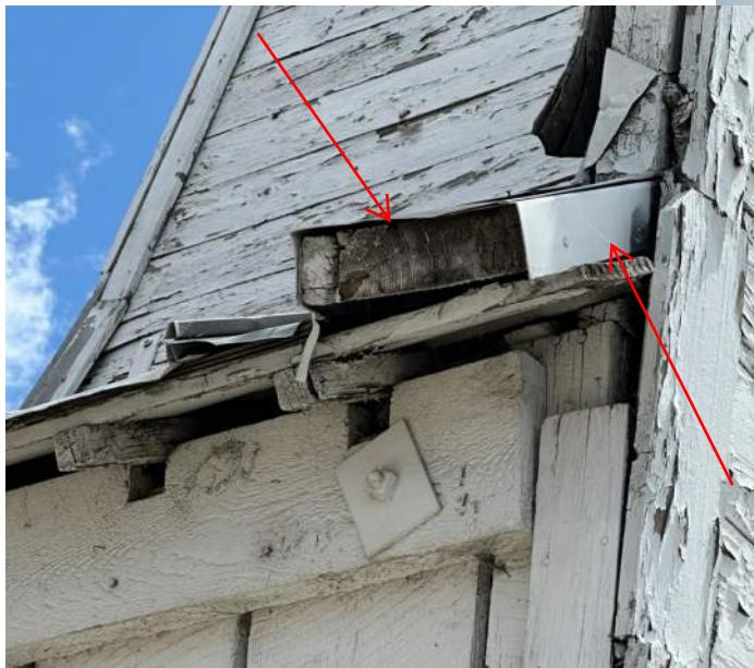
South backside of west facade with plywood, cantilevered exposed board, and missing wall flashing at roof
