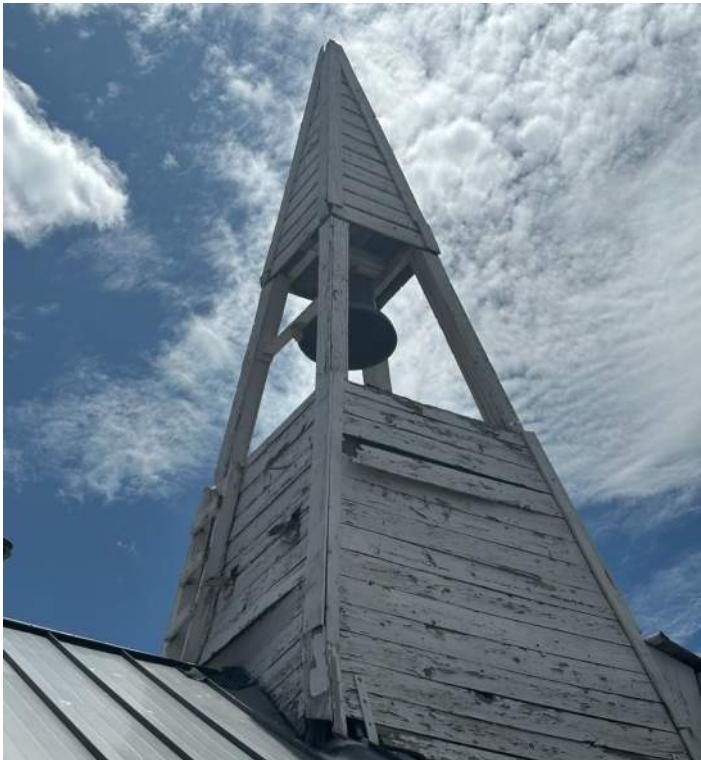
Bell tower view from northeast. Note loose and warped siding
