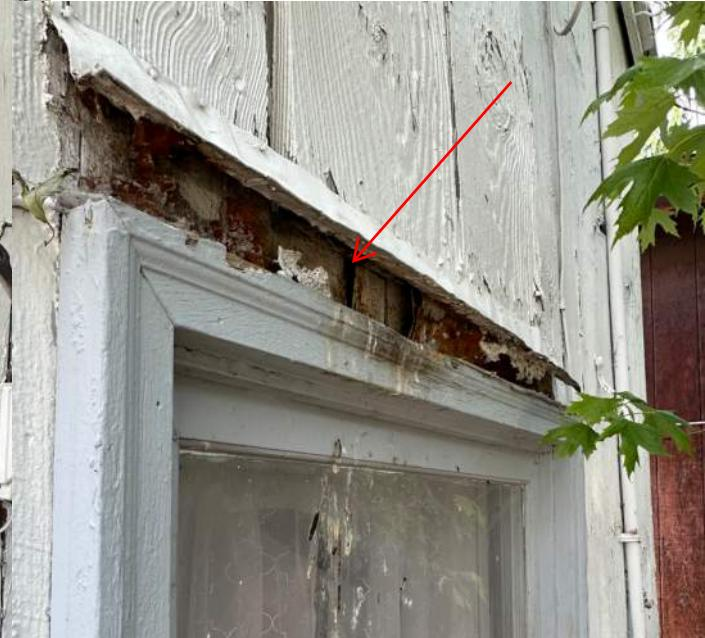
Northeast window at header with old flashing, and missing trim board
