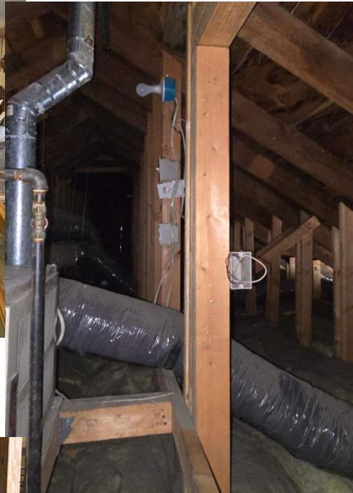
Attic with new structural framing, ductwork, and HVAC unit on right
