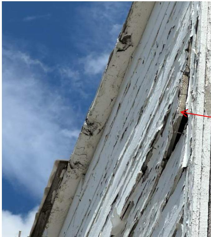
West facade with loose and warped siding
