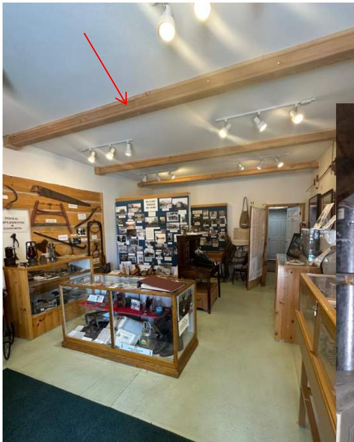
Museum interior with new glulam beam structural beam exposed
