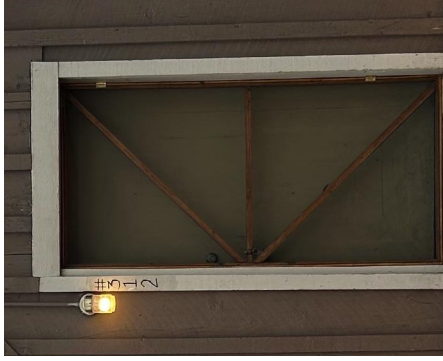
REPLACEMENT FOR NON-COMPLIANT EXPOSED BULB
