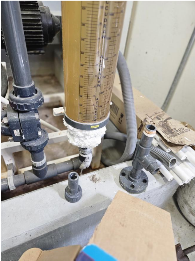
Figure 1: Work Item 8: Existing piping that will be replaced, evidence of chemical leaks
