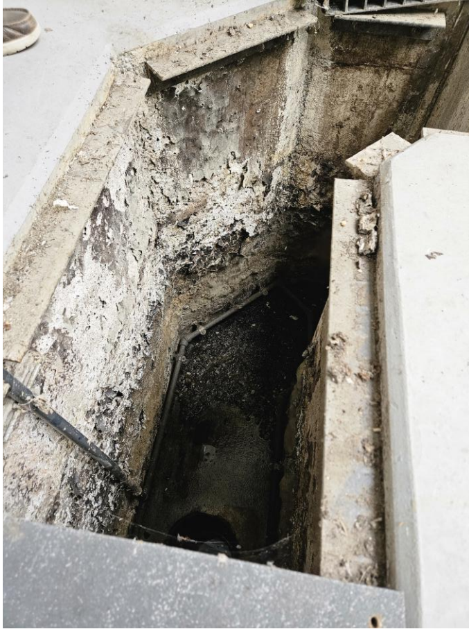
Figure 7- Headworks channel surface damage
