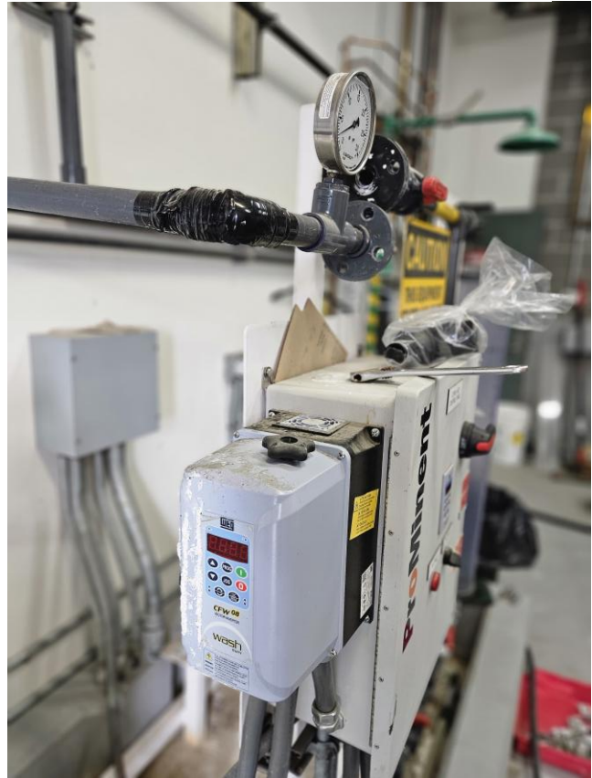
Figure 1: Work Item 8: Existing piping that will be replaced, evidence of chemical leaks
