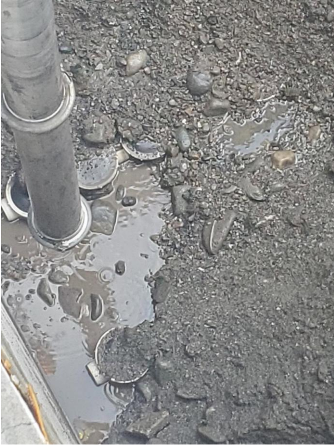
Figure 2: Item 12- Aeration Basins before and during cleaning
