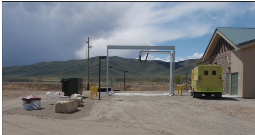
FIGURE 5-6: LIQUID SLUDGE HAULING
