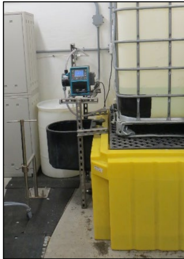
FIGURE 5-4: EXAMPLE SODIUM HYPOCHLORITE FEED SYSTEM
