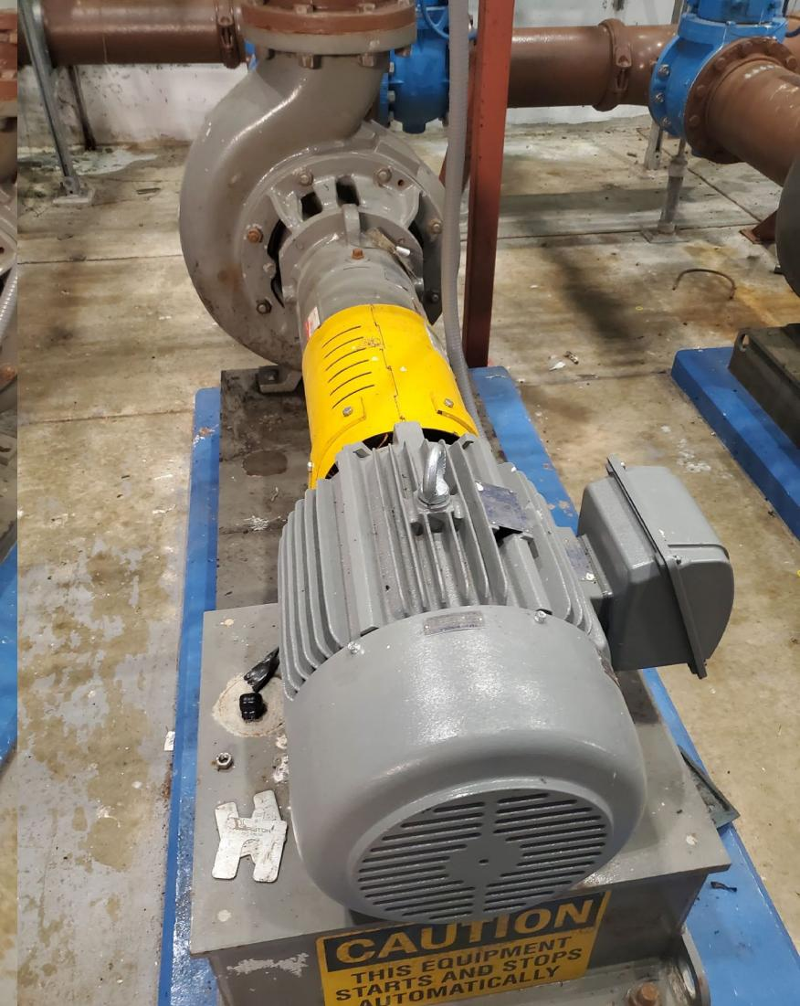
Primary pumps rebuilt or replaced.
