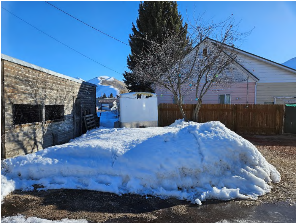
Alley Near Northwest Corner of Lot 6, Block 24 (Shed Encroachment)
