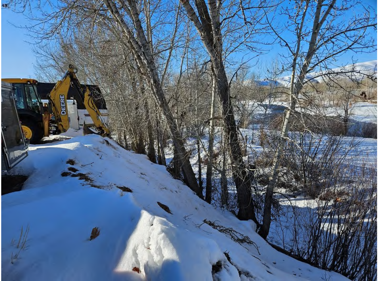
Northern Property Line @ Top of Bank of Proposed Lot 3A (Walnut Street) Facing South
